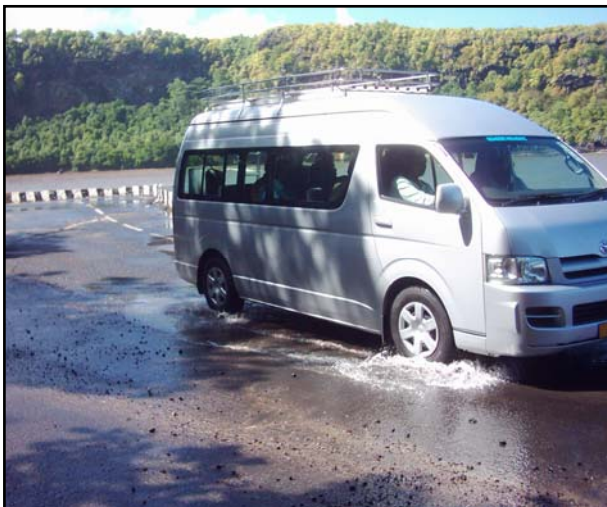
Flooded coastal road at Lardier
