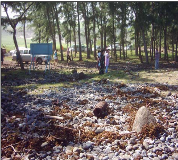
Gabion stones used to protect the beaches against high waves projected 60 metres off the high water mark
